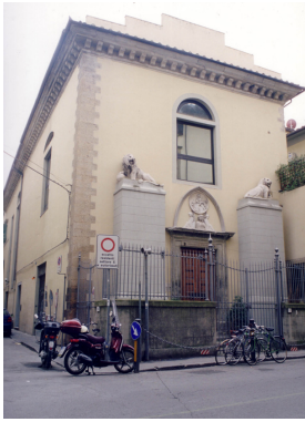
Figure 2 - Exterior of Santa Chiara from Via dei Serragli, Florence, 2008. Photograph: Donal Cooper
